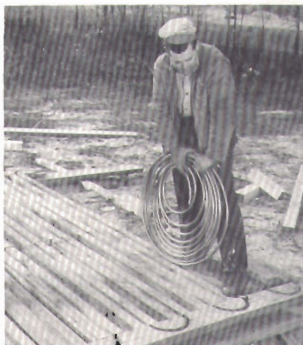
A wooden form, or mold, is quickly constructed, in sections easily moved from job to job. The workman, with a section of coiled soft copper tube starts the simple operation.
